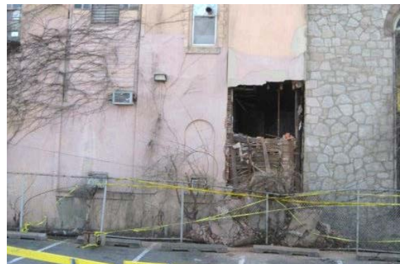
North side of church with annex to left and main church to right. Note rectangular hole in the annex on the lower right side due to partial collapse. Below is a blow-up.
