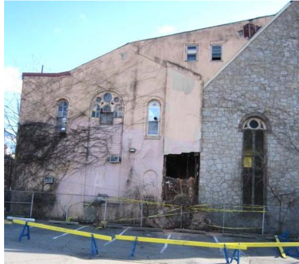
North side of church with annex to left and main church to right. Note rectangular hole in the annex on the lower right side due to partial collapse. Below is a blow-up.
