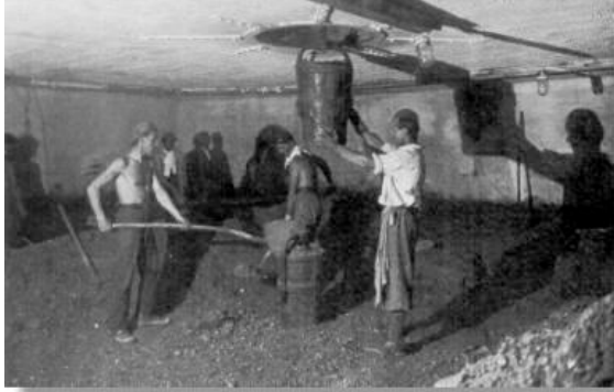
A photo of the work inside the caisson. It was hot and humid and had a distinct stench
