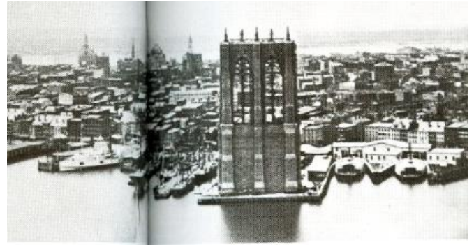
photo of the nearly completed Manhattan tower. East River in foreground, Hudson River in the background
